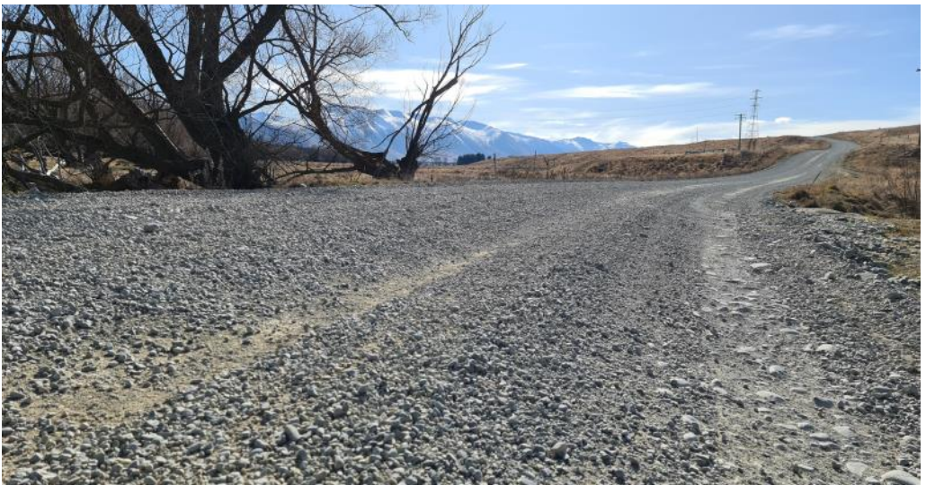
An uphill view of the troublesome corner on Quailburn Rd
